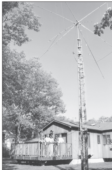
Fig 14-1— Showing a stealth antenna is easy—you show the sky. Rather than just the sky, here's the view at K2UO's QTH showing his low-profile 10/15/20-meter quad and his beautiful home in a wooded residential area in New Jersey. With his invisible 160-meter stealth dipole, George has worked 200+ countries on Topband.
